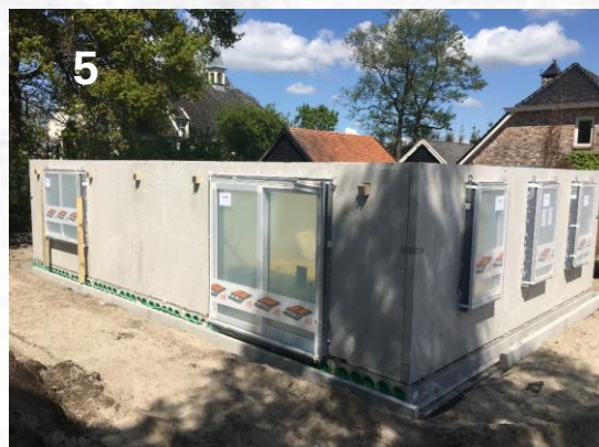
5 Setting up the wall elements on site...
