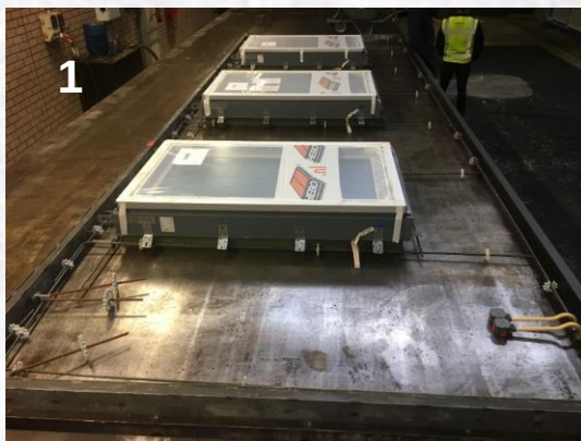
1 Prepare formwork with installation parts
