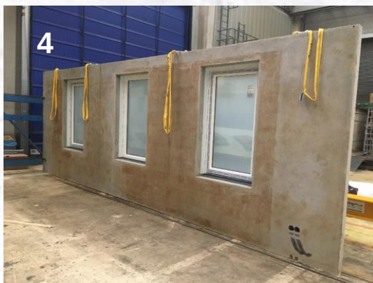
4 Strip the formwork and storage
