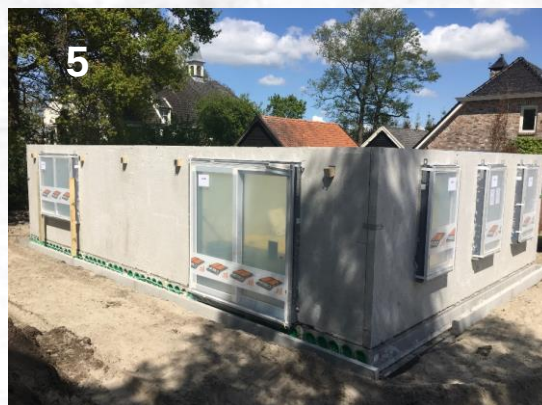
5 Setting up the wall elements on site...
